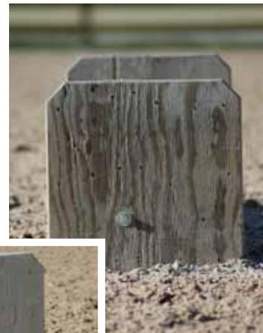
**ABOVE:** A lag bolt driven into the 4x4 from each end holds it in place. **LEFT:**
